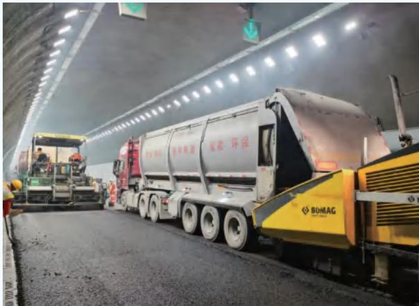
Pavement construction of Hangzhou-Huangshan Expressway applied dust-free waste collection equipment for the first time, reducing environmental pollution; it was the first large-scale successful application of an extremely thin wear layer in the province, while realising the quality (IRI pass rate of 92.5%), technology, and efficiency breakthroughs.
