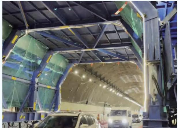
The Ningbo section in Ningbo-Taizhou-Wenzhou Expressway pioneered the development and application of intelligent and mobile maintenance cart, and achieved a breakthrough in the realisation of tunnel lining of the full cross-section and other maintenance of non-disruptive operations, reducing the impact on traffic.
